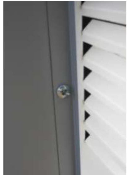
Step 23 screw in fixing bolts to connect heat pump module to storage tank
