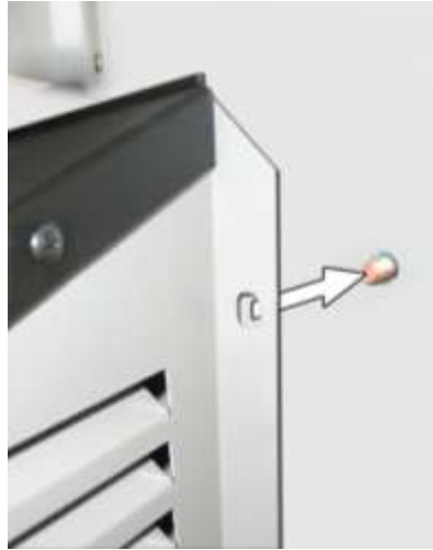
Steps 20 and 21 align heat pump module over studs and screw on flange nuts
