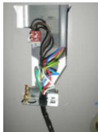
Step 3 withdraw the power cable
