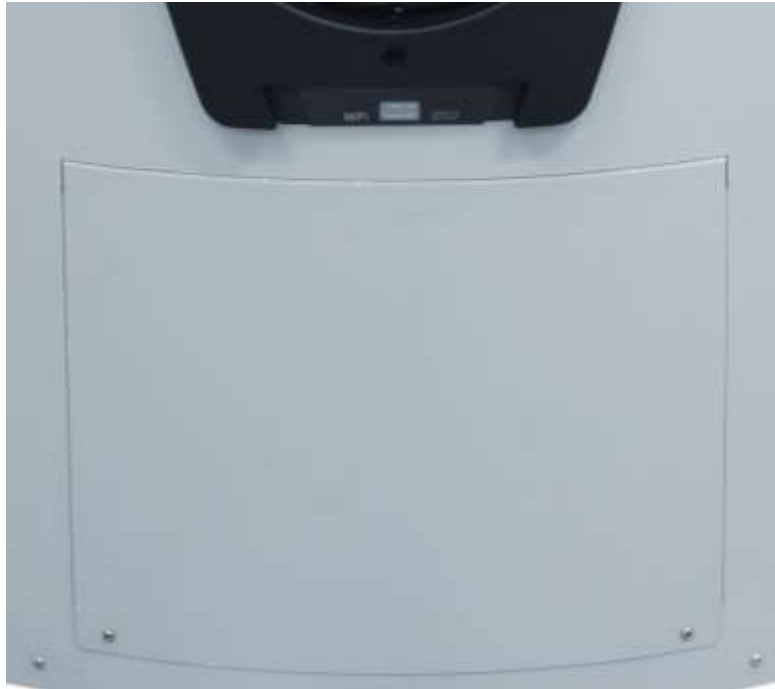
Step 29 replace heat pump module front cover
